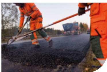
Construction materials and asphalt
